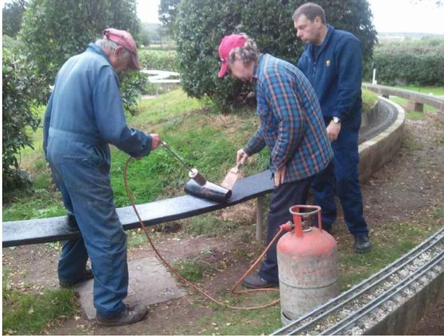
Laying roofing felt on the 32mm circuit—track laying next!
