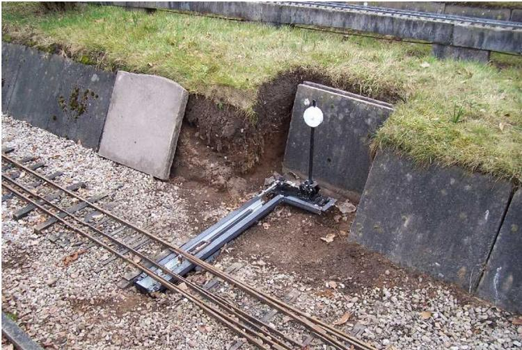
Completed new point mechanism at the station exit
